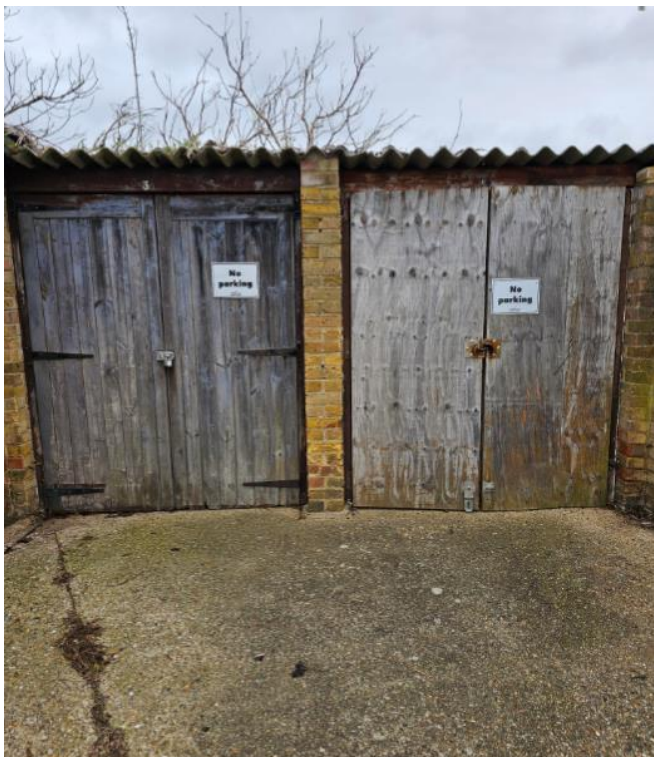
Figure 1: Photograph of sheds prior to their demolition.
