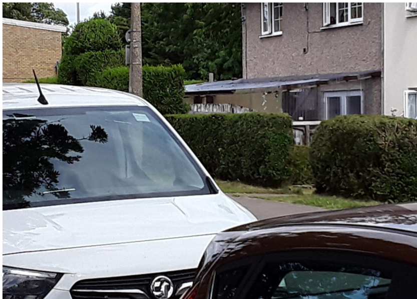
Figure 4: Existing front extension / porch which has been constructed at 134 Marymead Drive.
