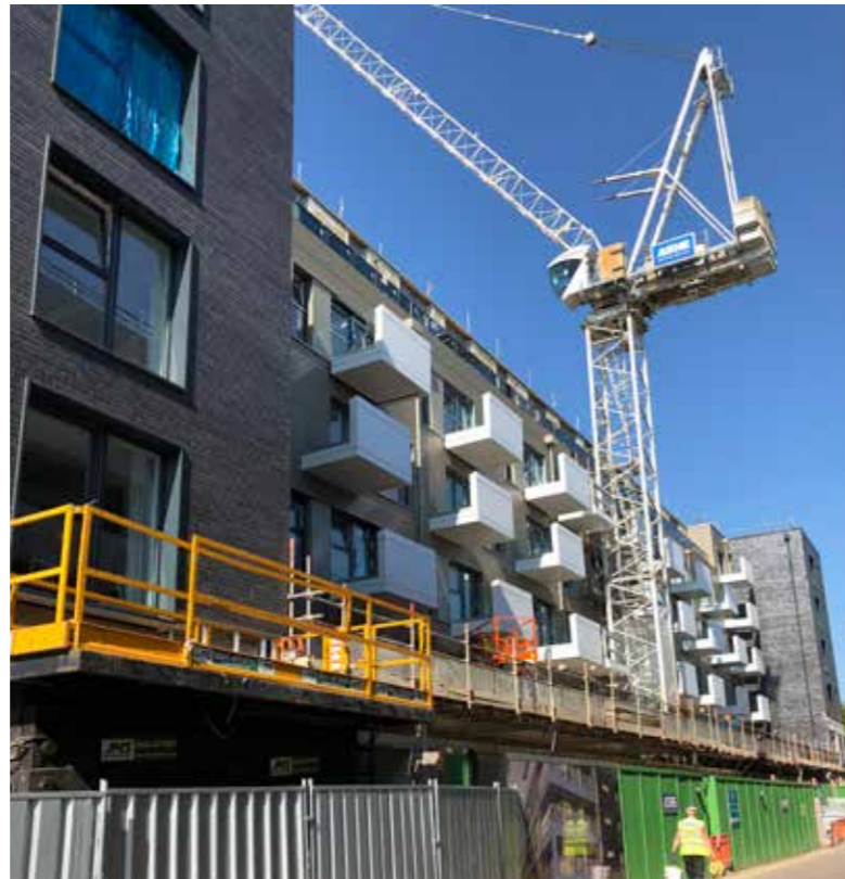
Figure 15: Construction work in Stevenage Town Centre
