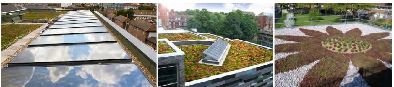
Figure 11 Examples of solar panels (l - © Viridian) and green roof options (c - © McLaw and r - © Langley Waterproofing) for flat roofs
