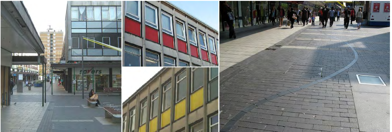
Figure 10 Timber clad canopies with steel supports (l), coloured pre cast panels (c) and block paving (r)
