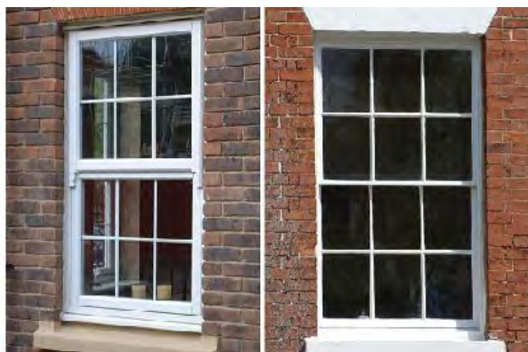
Figure 13 The uPVC alternatives, to the left of the example, are thicker, cruder frames.
