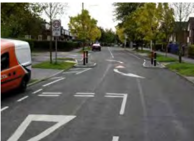
Figure 10 Examples of the traffic calming solution: pinch points
