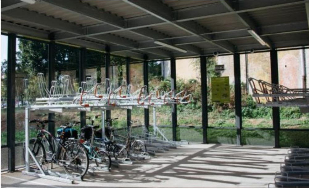
Figure 4. Example of a cycle hub interior
