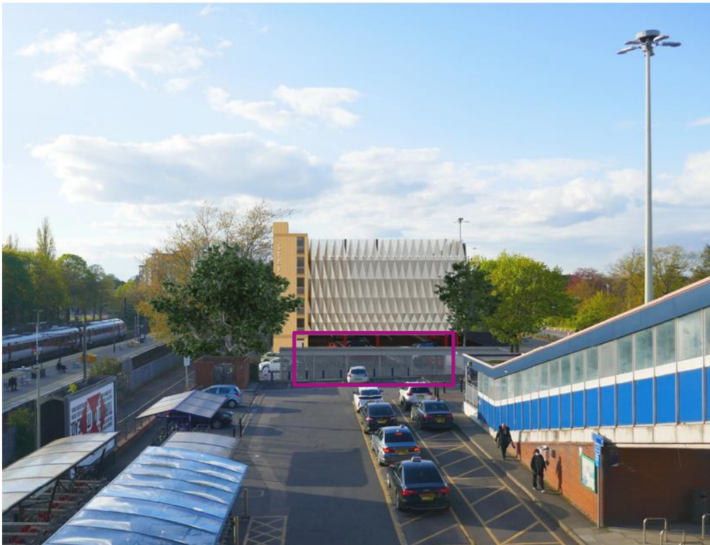
Figure 2. Visual from the station - South façade
