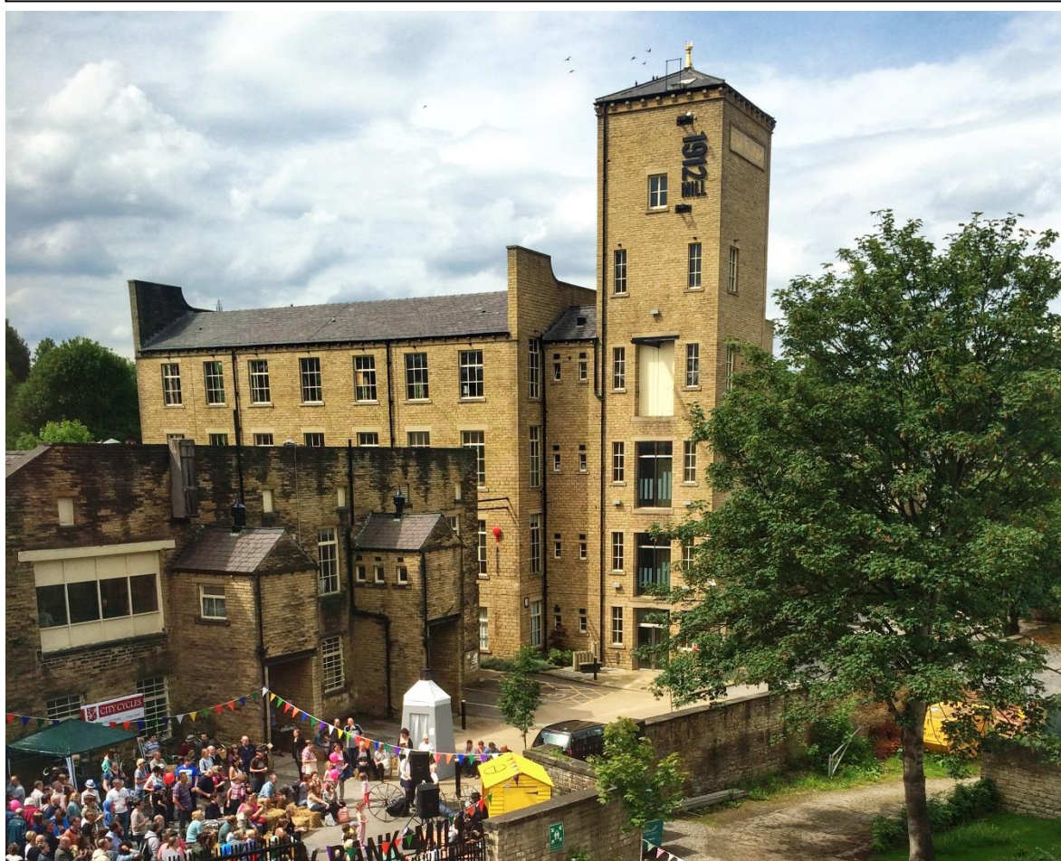
2 Sunny Bank Mills, Farsley, Leeds
